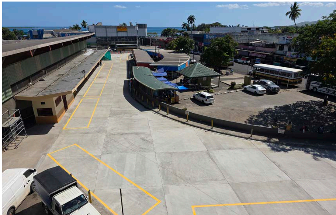
Image 12. Reconstruction of Lautoka City Bus Stand Pavement, Source: Lautoka City Council 2025
